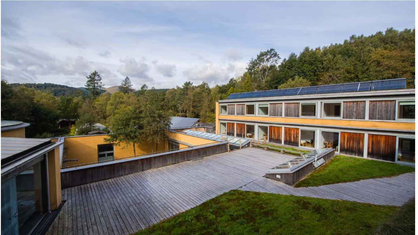
The WISE building, first floor deck
