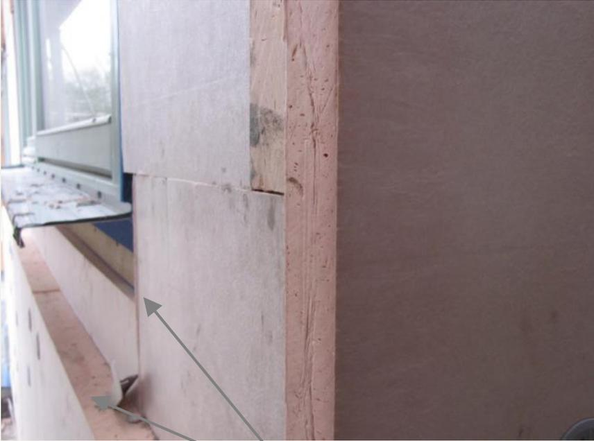
second layer of insulation overlaps timber sub-frame for windows
