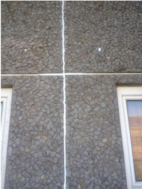
Airtightness jointing – Precast panels
